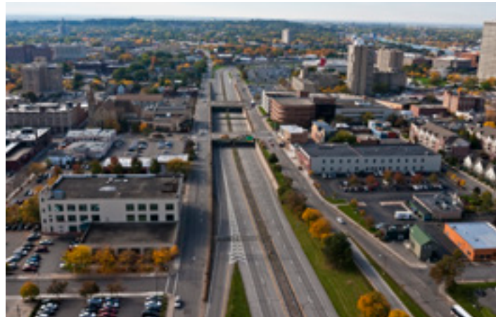
Rochester's Inner Loop, left, was built in the 1960s to encircle downtown. It divided neighborhoods and depressed property values while failing to deliver promised traffic benefits. In the last decade, the city decided to remove a portion and fill the highway trench, creating seven acres to be redeveloped and allowing new street connections for walking, biking and motoring. Building on that success, Rochester now plans to remove and redevelop an area more than twice the size.
