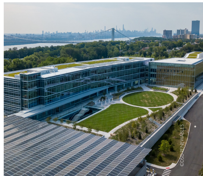
DSD's 1.3 MW solar installation for LG's New Jersey headquarters.
