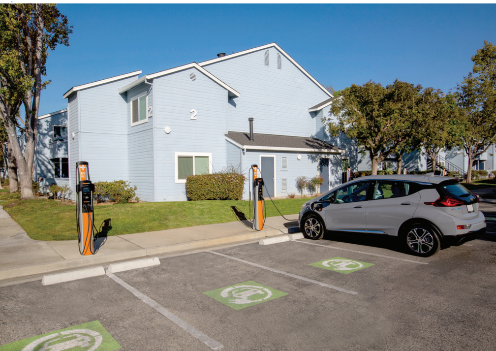
Today, the vast majority of personally owned EVs are charged at home in a driveway. More universal adoption will also require access to charging in multifamily situations such as the one above.
