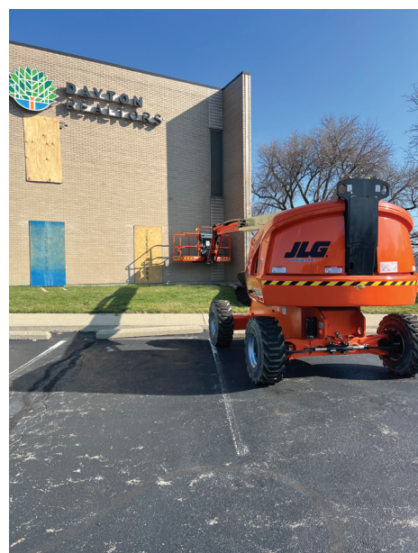
Dayton REALTORS® is renovating its 1980s-era building.
