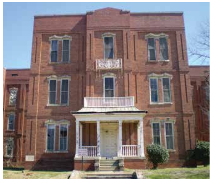
THE OLD WALKER BUILDING PRIOR TO RENOVATION
