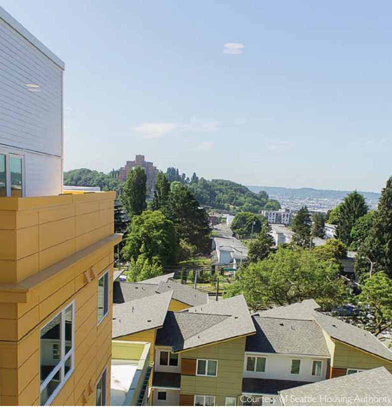
Courtesy of Seattle Housing Authority
