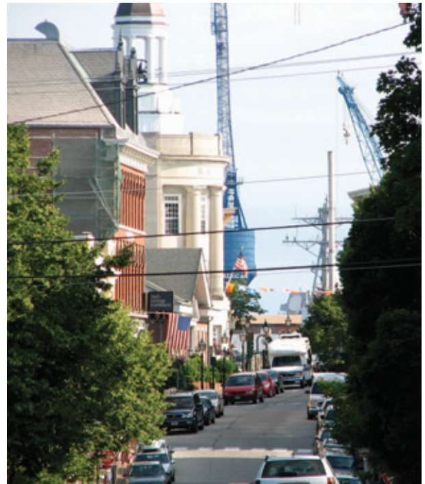
(Below) Artisan, one of the buildings participating in the CDBG Facade Master Plan project, underwent both a storefront rebuild as well as extensive interior rehabilitation. Home for more than 50 years to the local weekly newspaper, The Woodbine Twiner; it now houses a cooperative gallery and art education space including a glass hot shop in the rear annex. The Twiner moved to a smaller, more efficient office suite two doors down.
