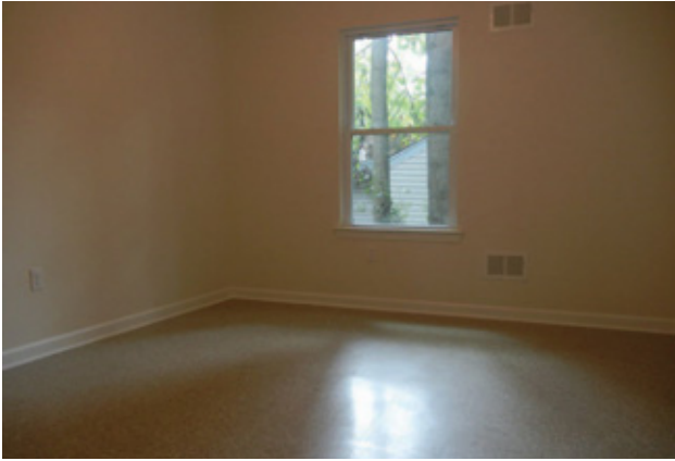
Interior of Community Options' house after remodeling
