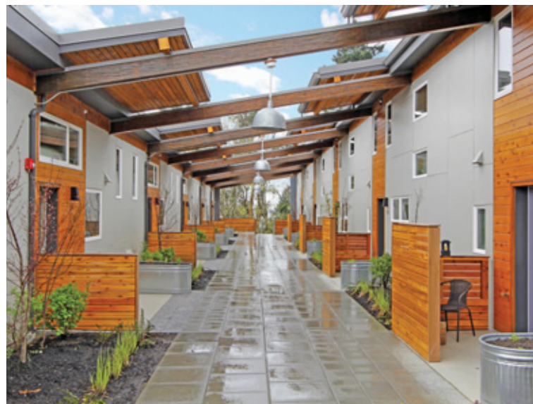
Puyallup housing designed with the longhouse theme in Tacoma, Wash.
